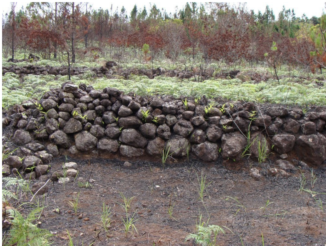
Fig. 7 – Retaining wall constructed as part of a horticultural terrace, site KKR003, Isle of Pines (photo L. Lagarde, 2010).
