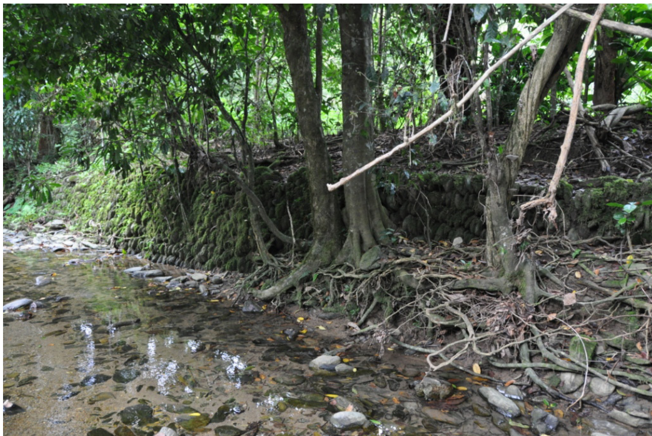
Fig. 11 – Example of retaining wall of a river bank, Hienghène region.
